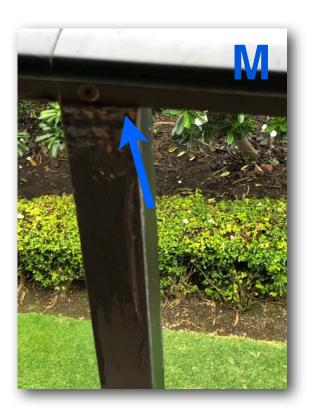
Areas of corrosion on railing
