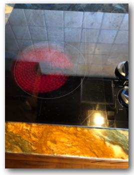
The left front range burner is functioning, but is offset by inches under the rangetop glass. It's unclear whether this is a manufacturing defect or a usage/installation defect where the element has shifted.
