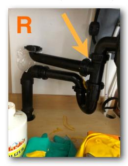
The sink installed is single bowl with disposal, yet there is an extra drain for a double bowl sink that could leak during a clog and cause damage. The T joint can be removed and an extension tailstock installed.
