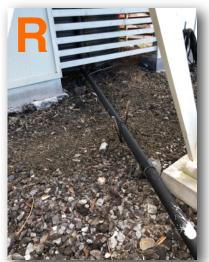
This 3" pipe is for filling the catchment tank in times of low water from a water truck on the street. The pipe span is largely unsupported, balanced on rocks and pipe could break during an emergency fill.
