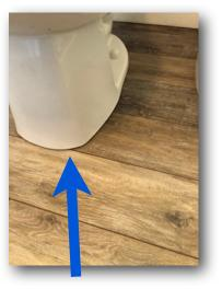
Toilet Base could be sealed to prevent moisture going under base and to provide stabilization.
