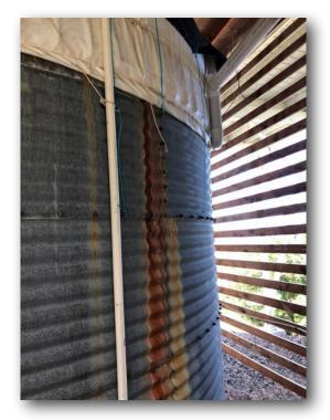
Minor Rusting on the water tank. Typical from poorly functioning overflow
