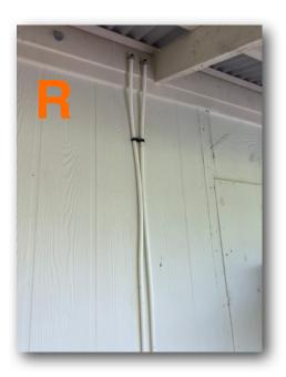
PEX piping on exterior for the outdoor shower could be painted for UV protection.
