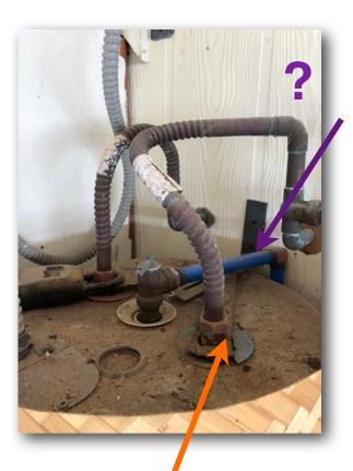
Potential Leak: Cold water inlet pipe nipple on water heater is heavily rusted
