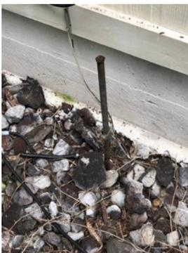
Double Grounding Rods spaced 6 feet (around corner)
